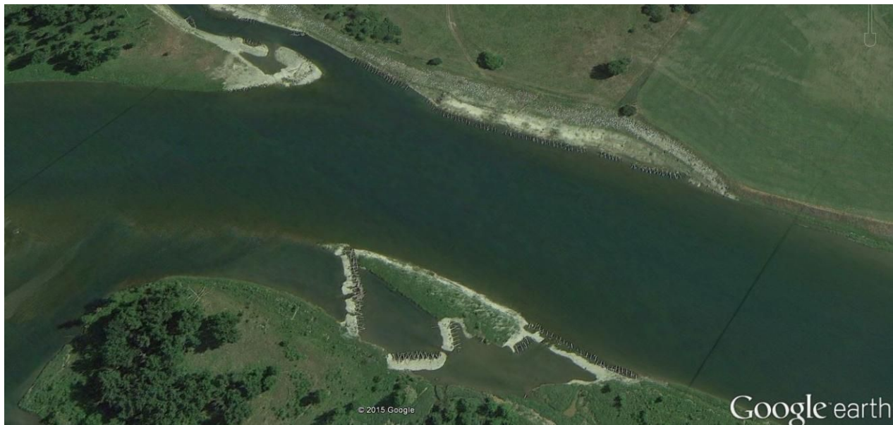
Figure 6. Examples from the Kootenai River, Idaho, USA, of wood pilings installed to create new floodplain areas to increase channel depth.
